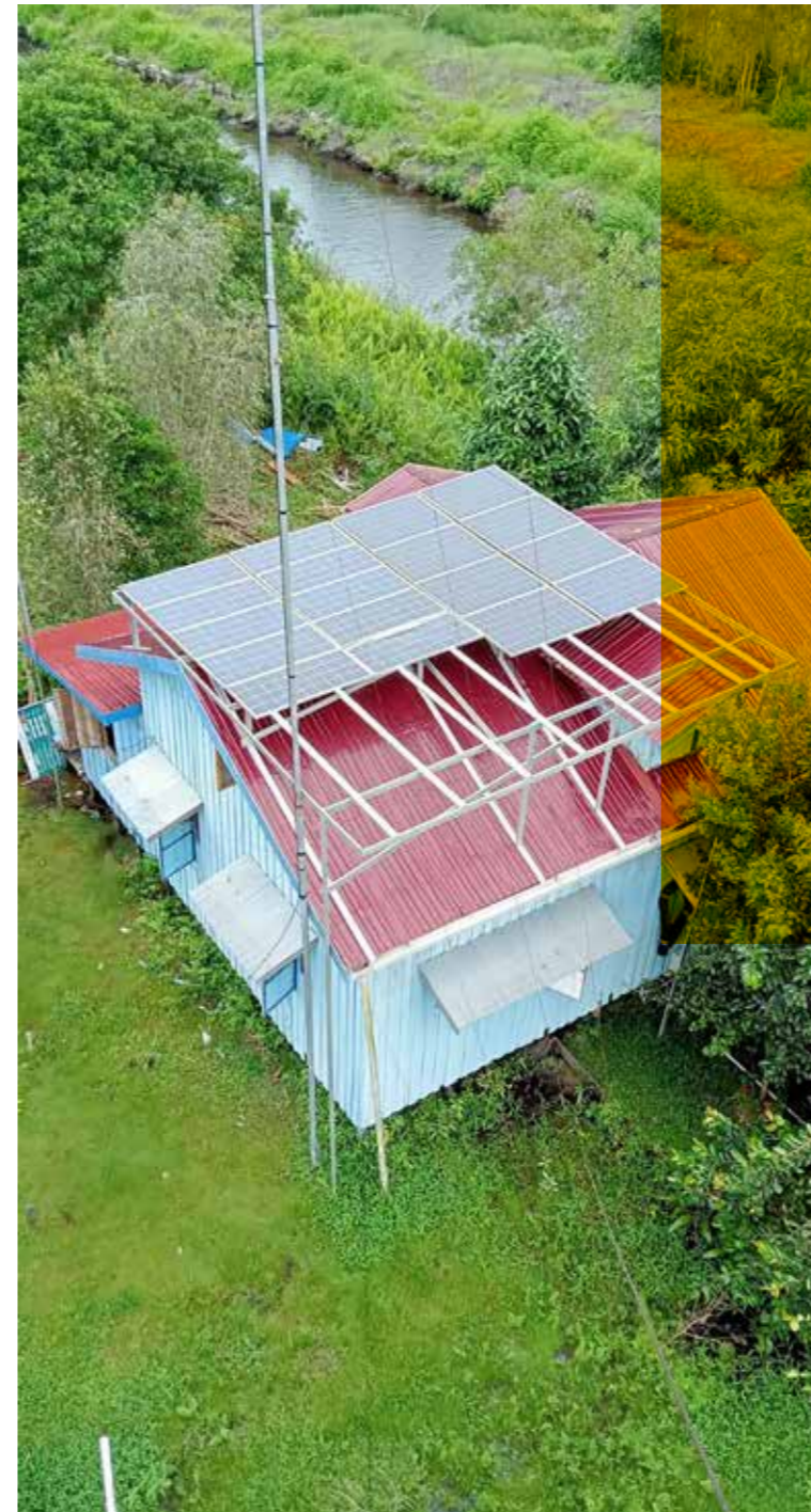
Installation of solar panels at Central Post
